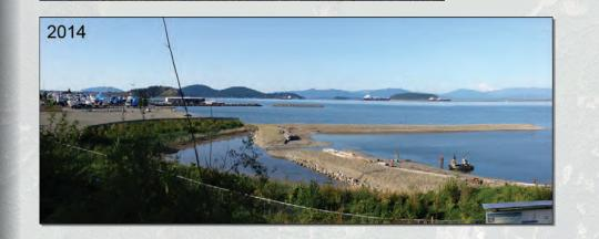
Cleanup at the former mill site included removal of 25,000 yards of soil and 52,000 yards of marine sediment. New habitat restored forage fish and salmonrearing shoreline. The final phase of cleanup is scheduled for 2020 to address low level dioxin contamination in the sub-tidal sediments.
