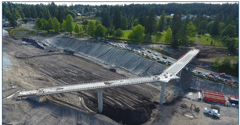
Photo 5: Point Defiance Trails Project during construction. Photo courtesy of Atkinson Construction.
