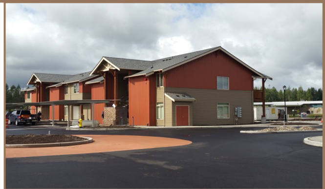
Puget Meadows West Apartments within the Meridian Campus received an NFA determination in the spring of 2017.
