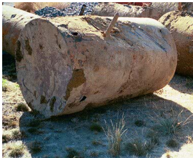
Figure 7-1: Removal of leaking underground storage tanks at Public Works facilities is a common use of Independent Remedial Action Grants.
