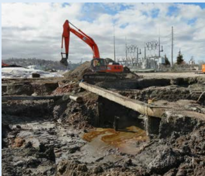
Figure 2 - K-C Site in 2013 during interim cleanup work
