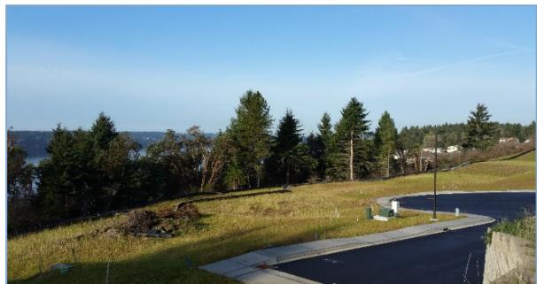
Photo 6: A cleaned residential lot is ready for development in Narrows Ridge
