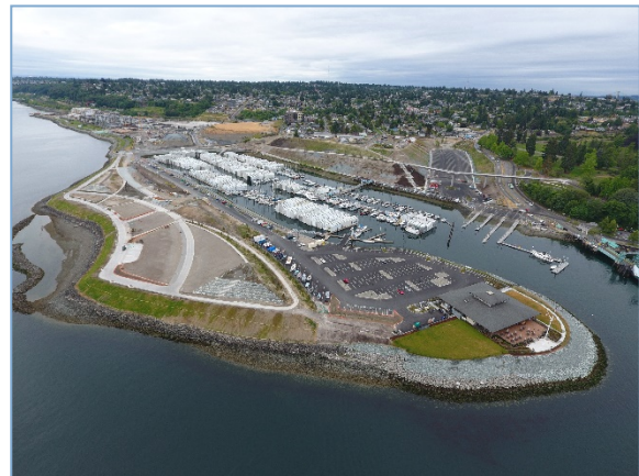
Photo 16: Point Defiance Trails project during construction. Photo courtesy of Atkinson Construction.
