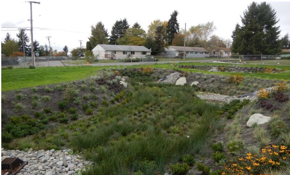
Figure 3. Sunset Terrace Regional Stormwater Facility bioretention cell provides enhanced treatment for 2.9 acres. Photo Credit: City of Renton
