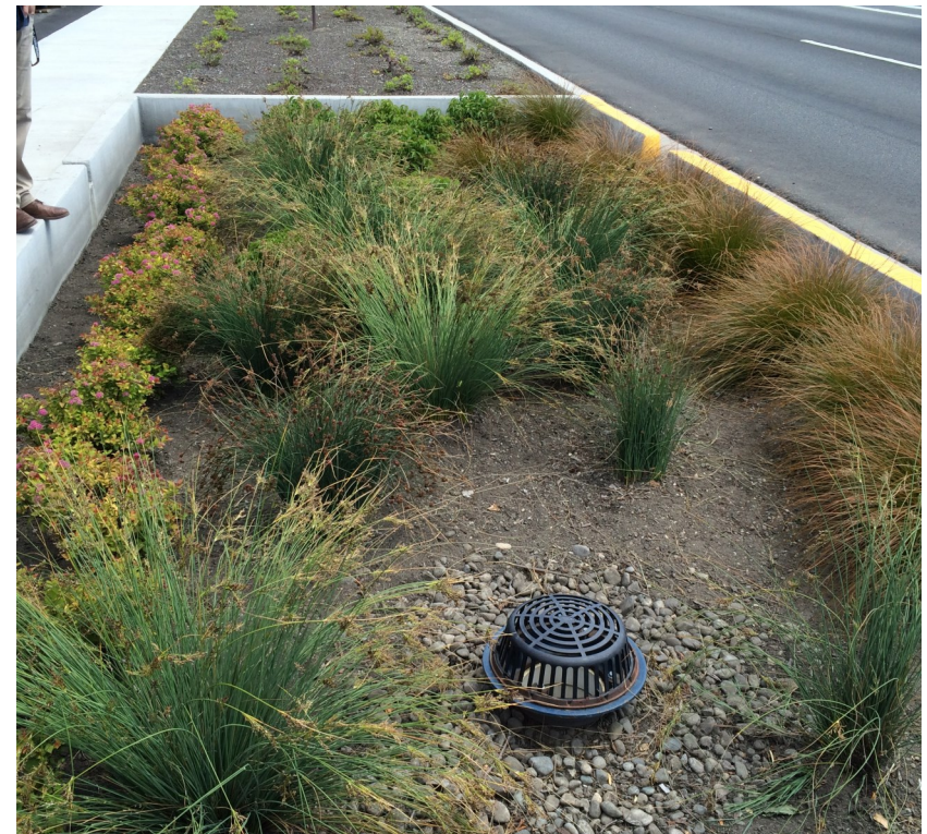
Figure 19. Bioretention facility in the City of Longview.
