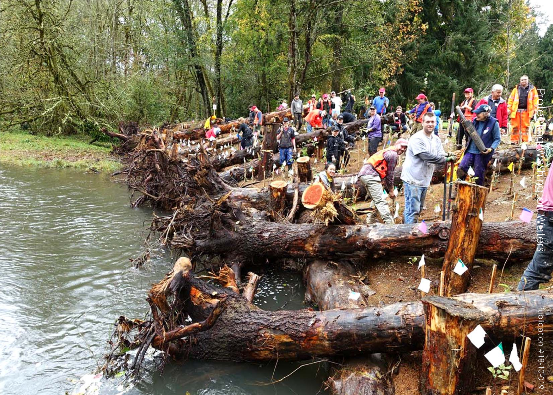
Figure 10. Clark Public Utility District recruited volunteers from the community to help restore Salmon Creek. Large woody debris (LWD) helps stabilize streambanks, reduce sediment, and provide habitat. Photo Credit: Clark Public Utility District
