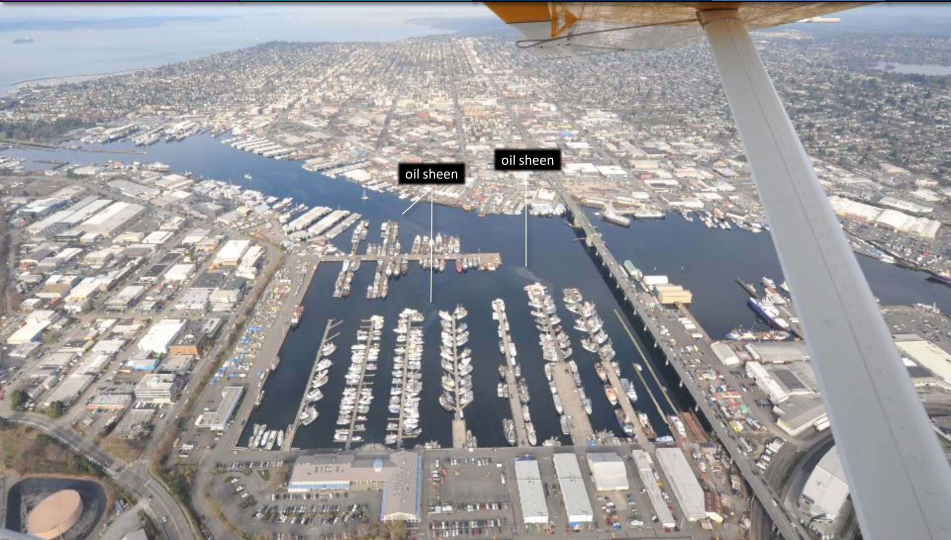
Repeated oil sheen on water near Seattle Fire Station, Dock 3. Location: Salmon Bay, Seattle (Central Sound), 2:25 PM
