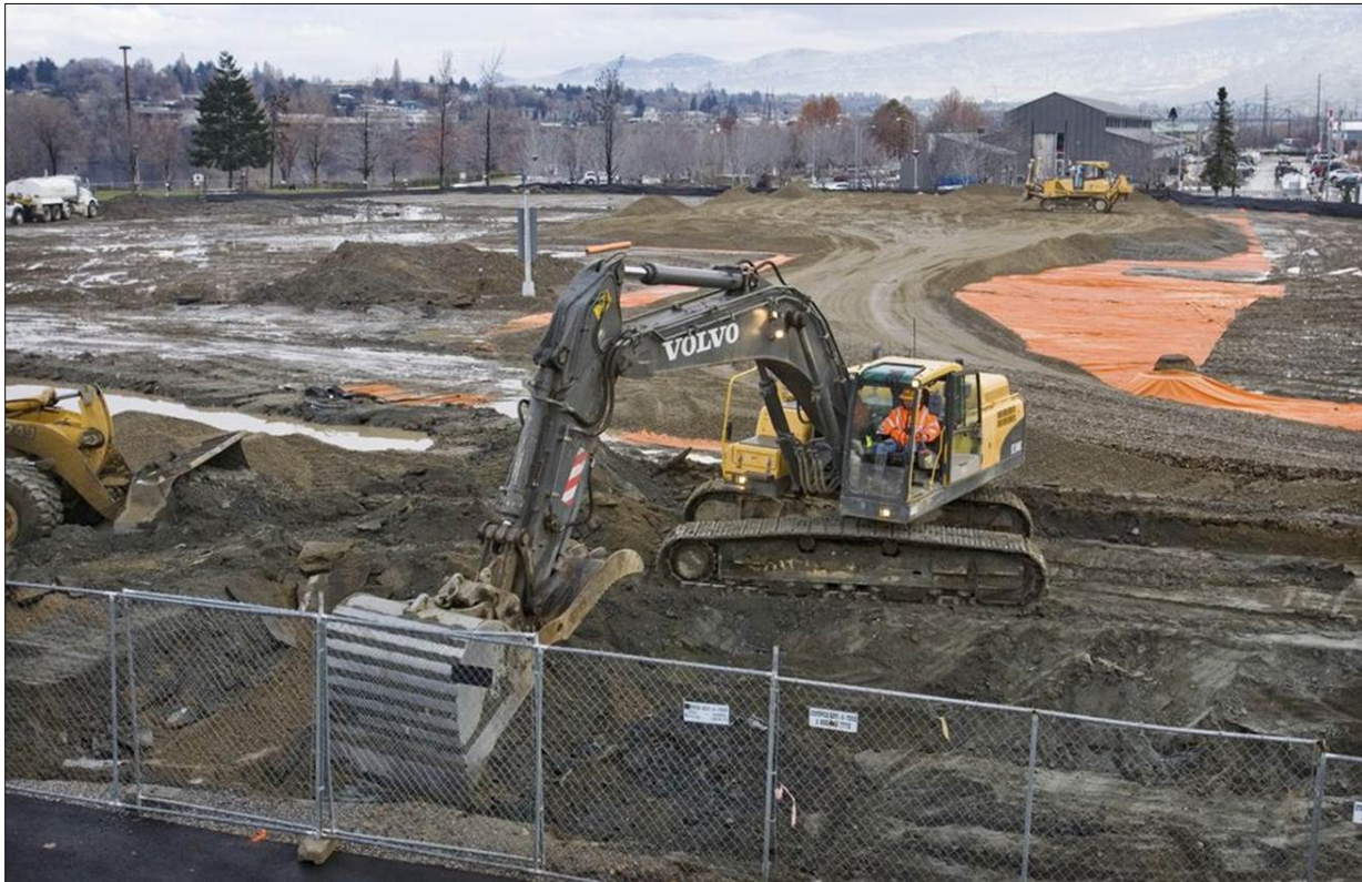
Figure 37: Before construction could begin on the new Wenatchee hotel, cleanup contractors removed contaminated soil from the site, then capped it with a foundation of the new building footprint, parking lot, and landscaping. An Environmental Covenant was recorded for the property to ensure the cap remains in place. Photo credit: Washington State Department of Ecology, 2015.
