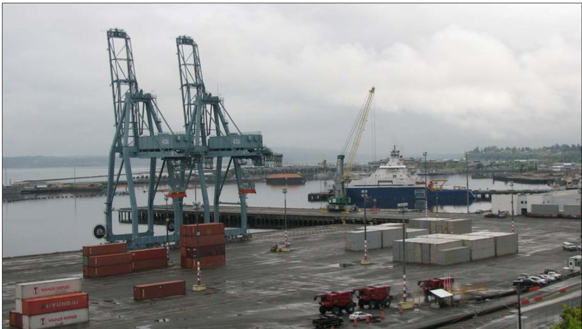
Figure 1: Pacific Terminal and cranes at the former Weyerhaeuser Mill A site at the Port of Everett. An interim action that removed contaminated sediment from the in-water environment allowed the Port to move forward with a marine terminal enhancement, resulting in improved navigational access to Pacific Terminal. Read the story on p. 143. Photo credit: Andy Kallus, Washington State Department of Ecology (2013)
