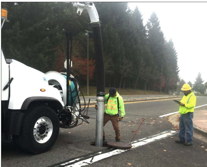
Figure 34: City of DuPont staff clean and monitor catch basins using new tracking software. Photo credit: Washington State Department of Ecology
