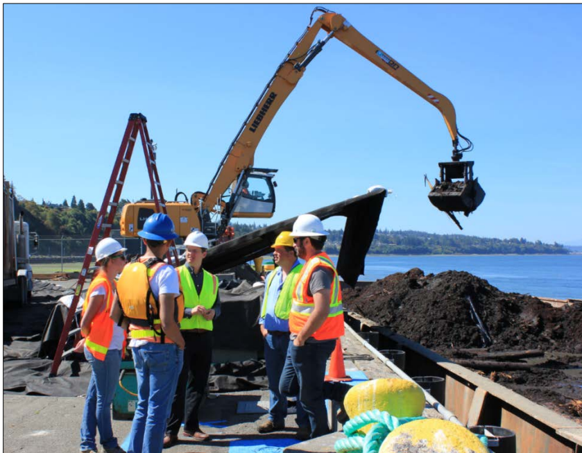
Figure 58: Coordinating efforts at the Port of Everett to offload contaminated sediment from barges to trucks for upland transport and disposal. CSID 2146 . Photo credit: Andy Kallus, Washington State Department of Ecology, 2016
