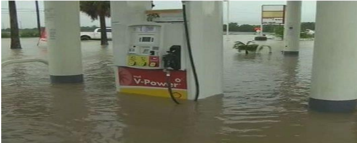
Service station flooded during extreme weather event.
