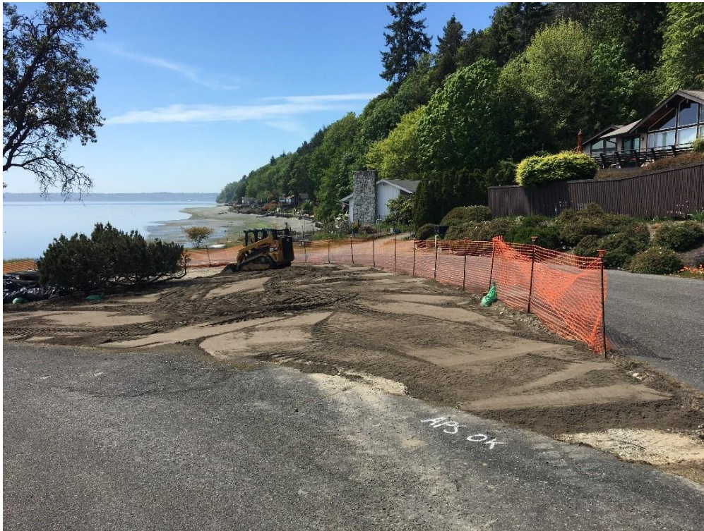
Figure 20: Sandy Shores Community Park undergoing soil replacement
