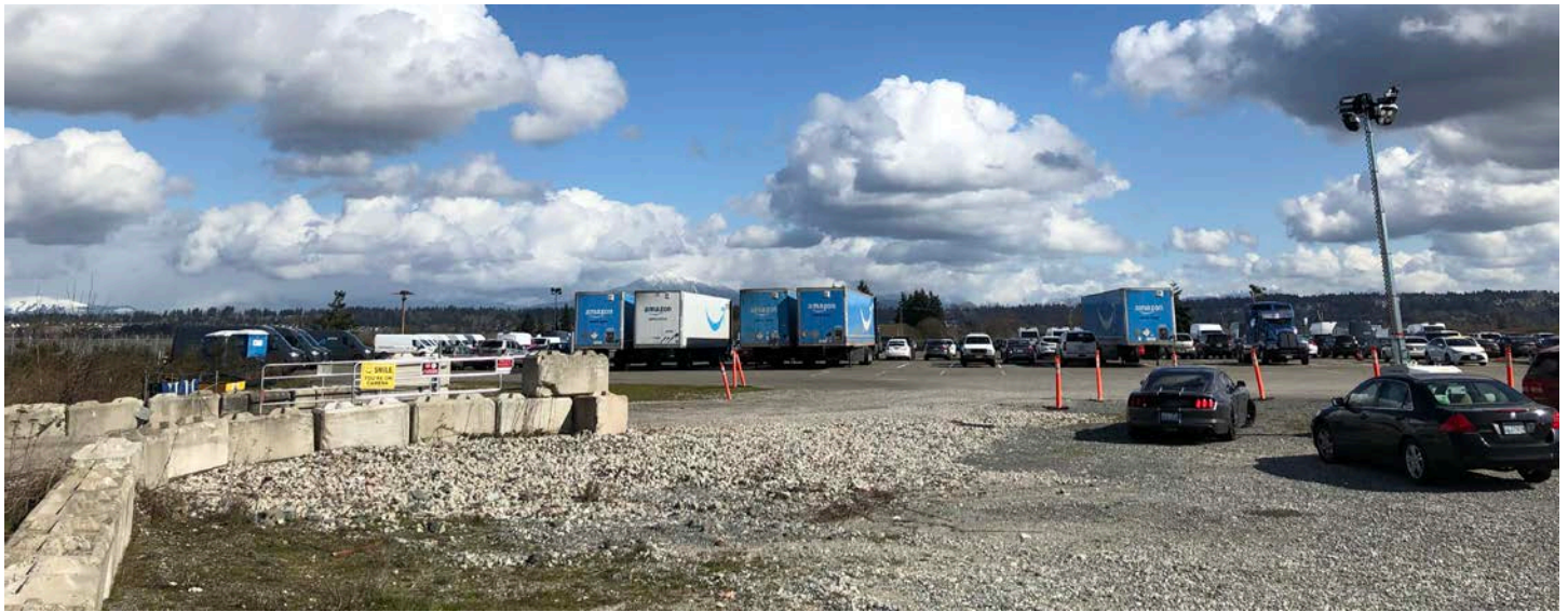
Cleanup site facing east, March 2020
