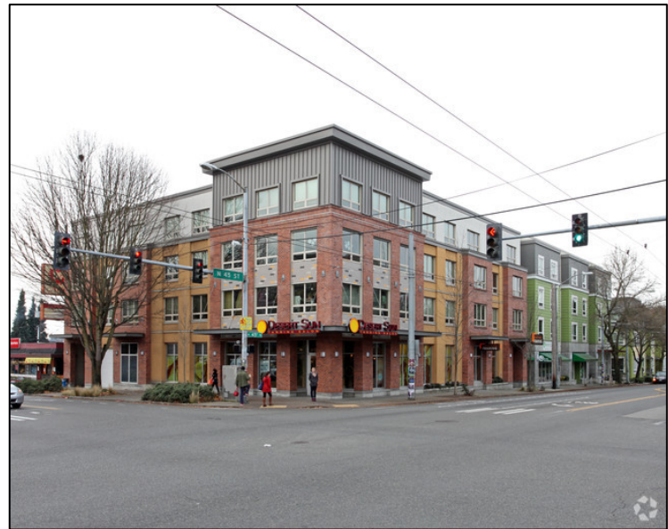
Stone Way Apartments
