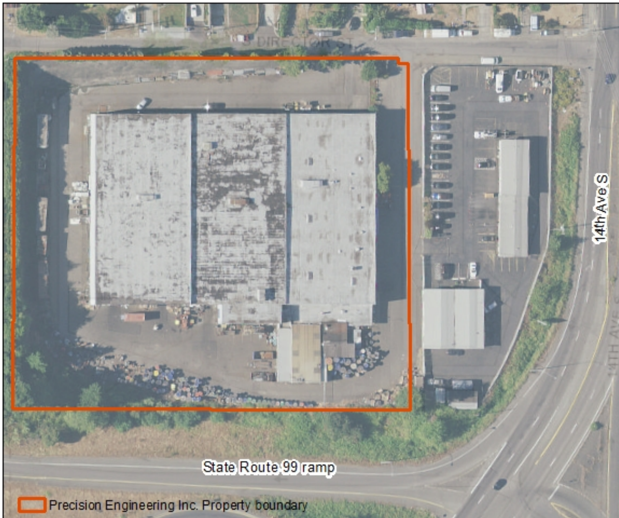
Aerial view of Precision Engineering Inc. Site.
