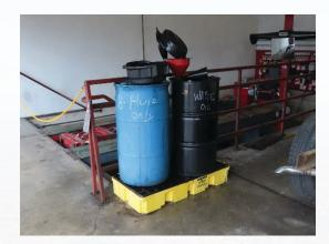
After: With secondary containment, the chances of the oil spilling to the stairs and needing to be cleaned up is reduced.
