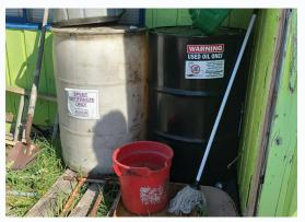
Before: Without secondary containment, any oil spilled during adding/removing materials from the drums would spill to the ground, causing soil contamination.
