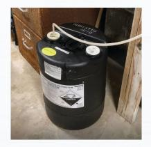
After: The new vapor-tight connector from the acid drum to the feed line.
