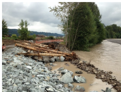
Engineered levy and logjams, resulting from good flood planning, are helping lower flood-related damages for the Pierce County town of Orting.
