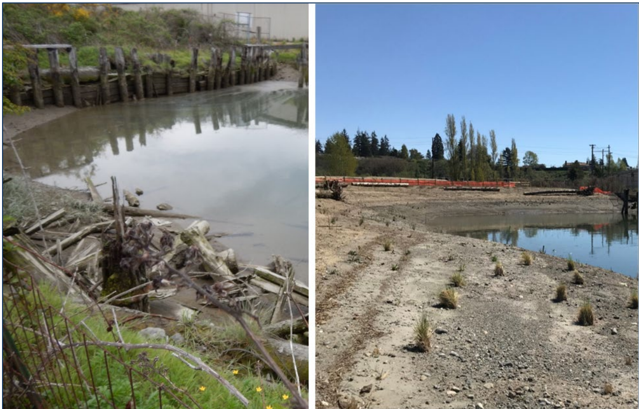
Figure 50 Before and after regrading the shoreline and installing habitat enhancements. Photo credit: Port of Everett Bay Wood Products site near Everett in Snohomish County. Cleanup Site ID 2581 (2019 and 2021)
