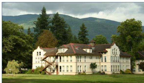
Figure 54: An Integrated Planning Grant awarded in 2014 galvanized the cleanup of an historical property in Sedro-Woolley that's now underway. Public participation and an Ecology remedial action grant during the 2019–21 biennium are helping the Skagit Valley community remove harmful contaminants from the soil and groundwater, and reimagine the multi-use site. (Ecology, CSID 10048 )
