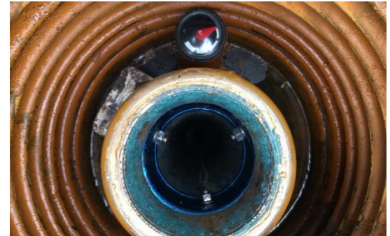
Double-Walled Spill Bucket with float sensor the 3-year test is required
