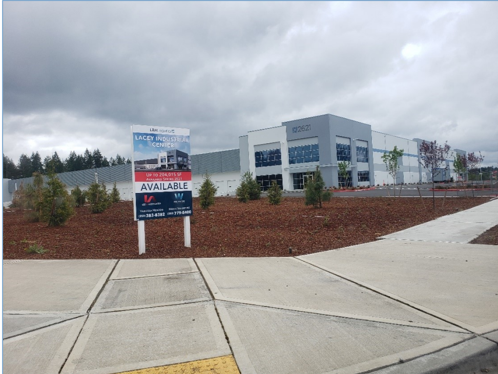
Figure 14: A completed Industrial Development at Lacey Construction on cleaned land
