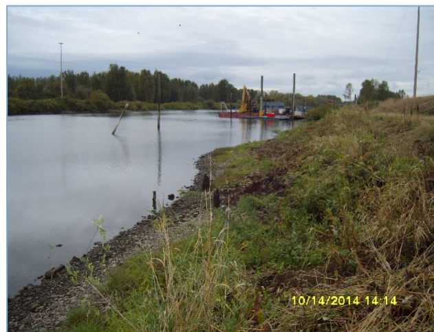
Figure 21: Lake River shore before rehabilitation
