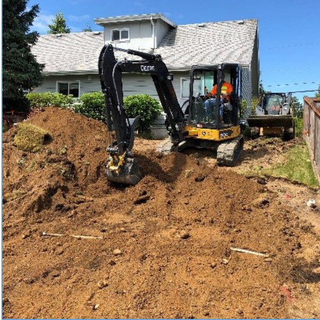
Figure 13: Contractors replacing soil in the backyard
