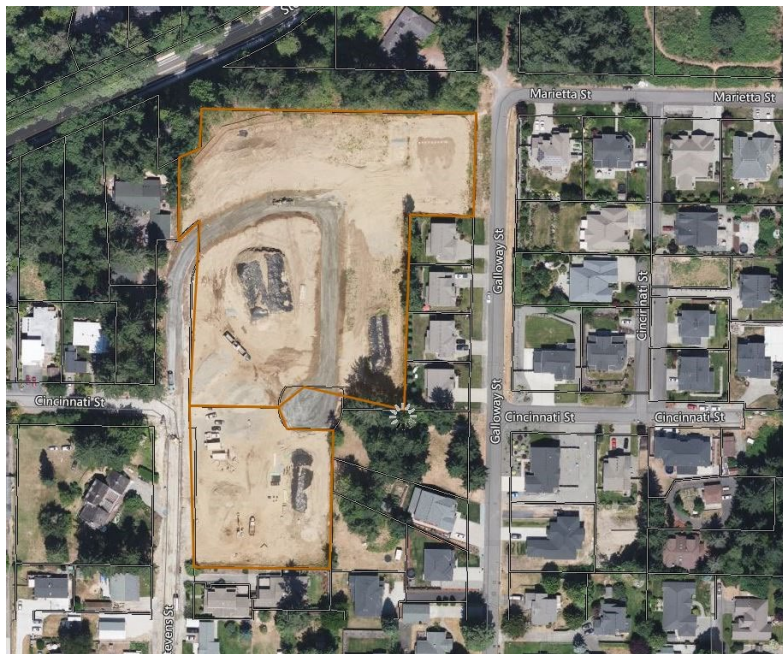
Figure 22: Norberg Estate after cleanup and development
