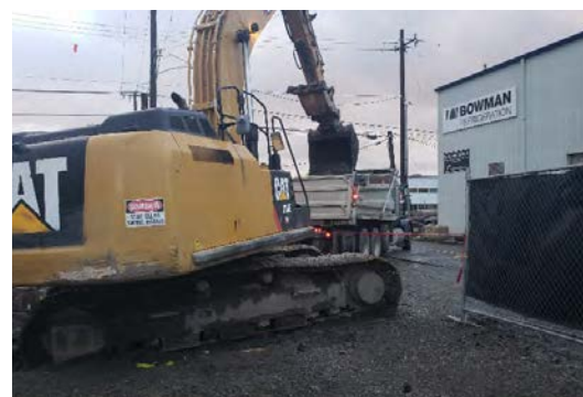
Removing contaminated soil from the site.
