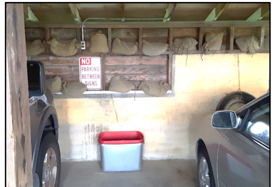
Mike stores filled sand bags on shelves and in nooks in his carport. Note the elevated electrical outlet above the sign.
