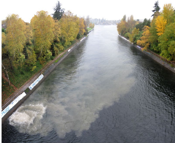
Montlake combined sewer overflow (Photo by Blake Feist).
