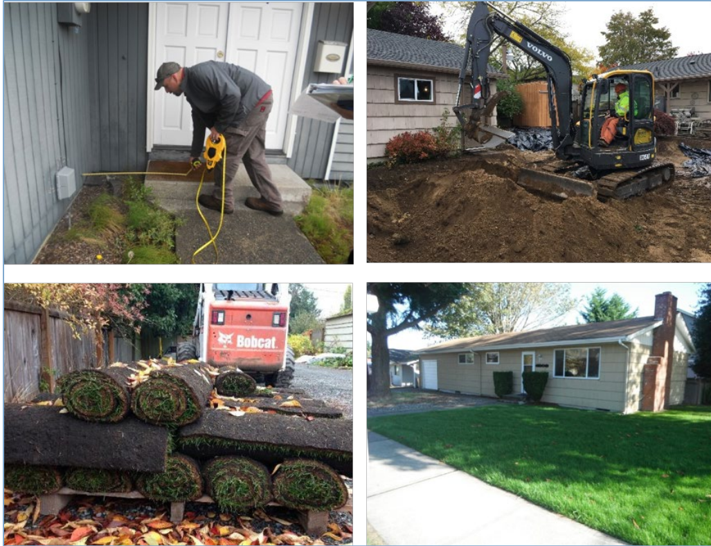
Figure 10: Steps towards soil replacement
