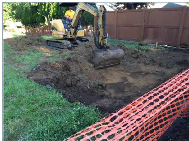
Figure 23: Soil replacement on a property
