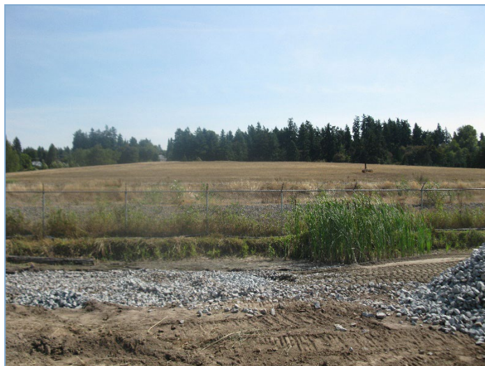
Figure 3: Landfill at the B&L Woodwaste site.
