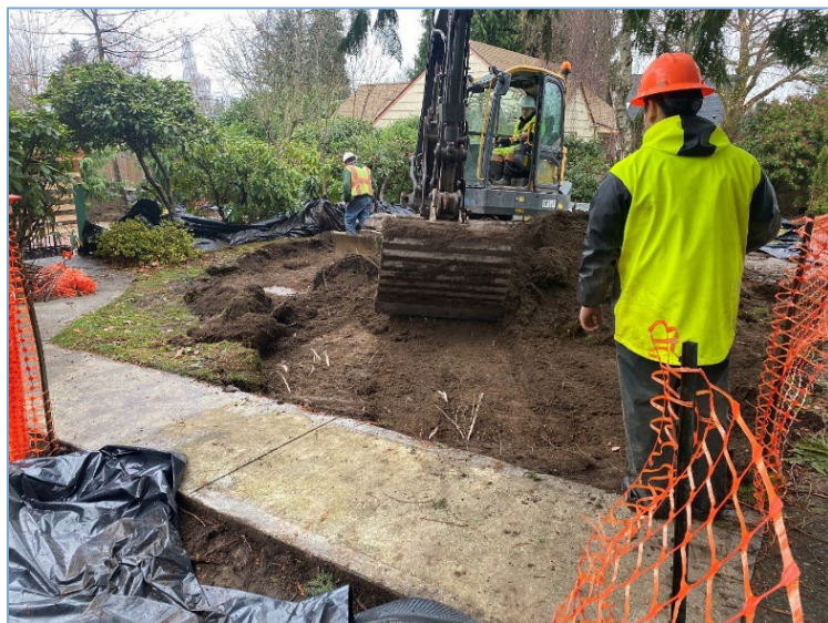
Figure 9: Soil replacement in progress
