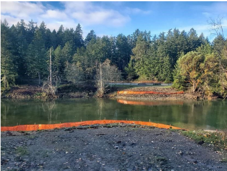
Figure 2: Removal of culverts to restore habitat at Milewah Creek
