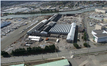
Aerial view of the cleanup site
