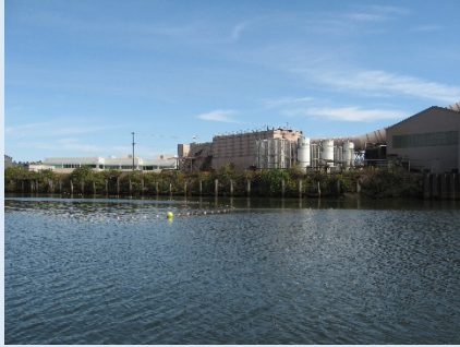
Jorgensen Forge Corp Cleanup Site from the Lower Duwamish Waterway
