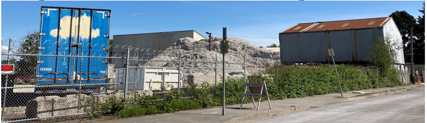
Northern portion of Independent Metals Plant 2 Cleanup Site
