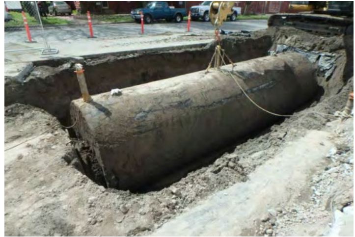
Underground storage tanks removed from the site
