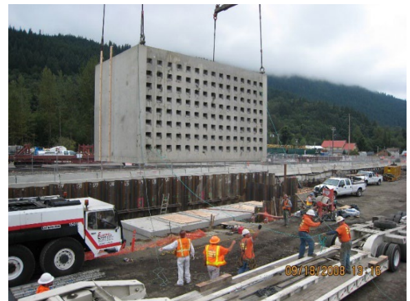
Installation of HCC treatment gate system, 2008
