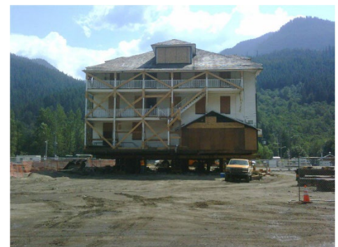
Temporarily moving the Skykomish Hotel, 2009
