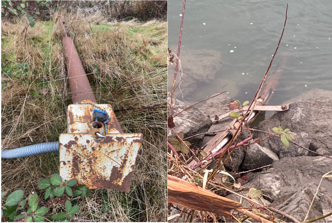
Figure 5. A slant pipe with anti-stilling windows at the Skagit River near Mt. Vernon (USGS Station ID 12200500).
