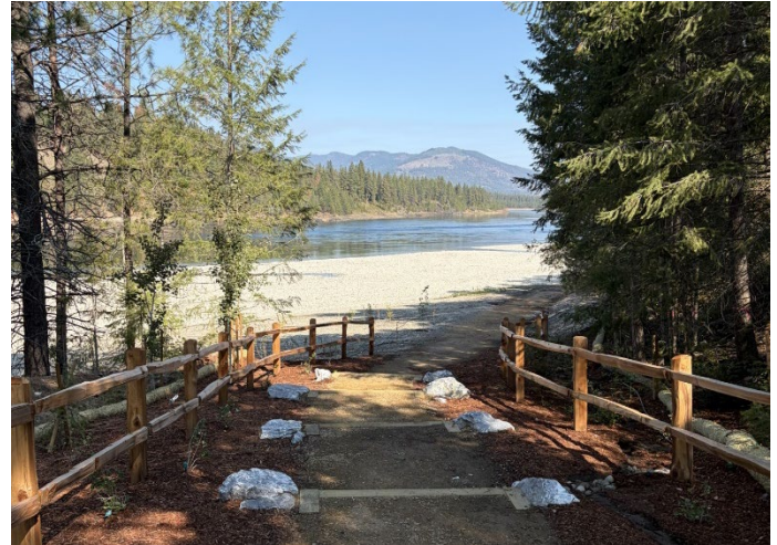
Hillside trail to the beach with stair steps and cedar fencing.
