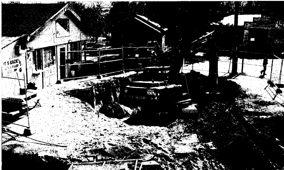
Soil is excavated from a leaking underground storage tank site at Arden's Country Store in Malott, Okanogan County.
