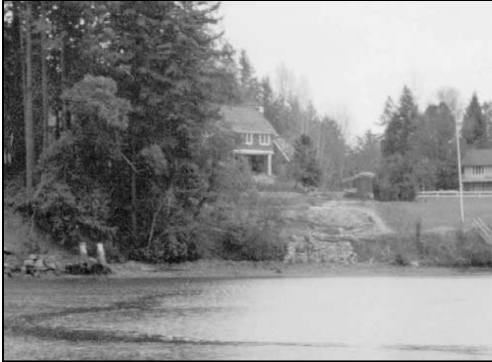
Figure 1. The Dick residence is sited well back from the water and trees north of the house were left. The riprap bulkhead on the north end of the site was installed by neighbors as an emergency measure prior to construction of the Dick's home (Photo: Jim Brennan).
