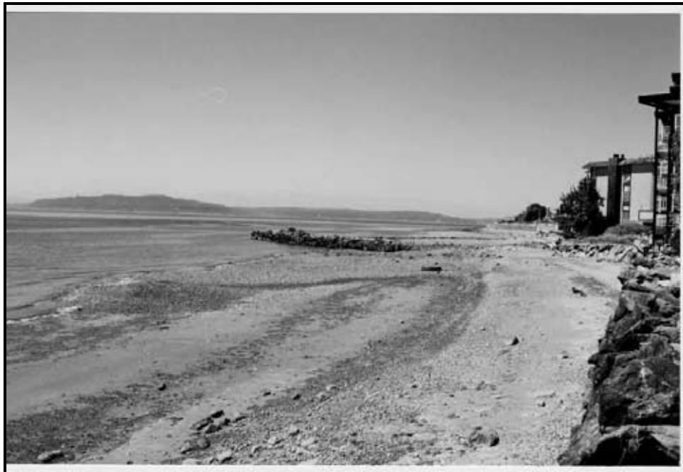
Figure 2. View to the north from 3701 Beach Drive, showing hardened shoreline and intrusion of bulkhead onto upper beach.
