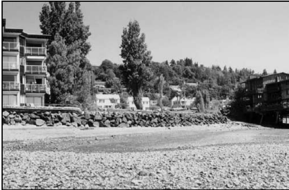
Figure 1. View of Cormorant Cove site from the beach at low tide. Much of the rock bulkhead will be removed when the project is constructed.
