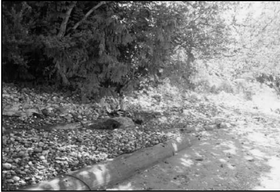
Figure 3. View southeast along beach shows anchored logs and added gravel. Compare to Figure 4 below of property to the north.
