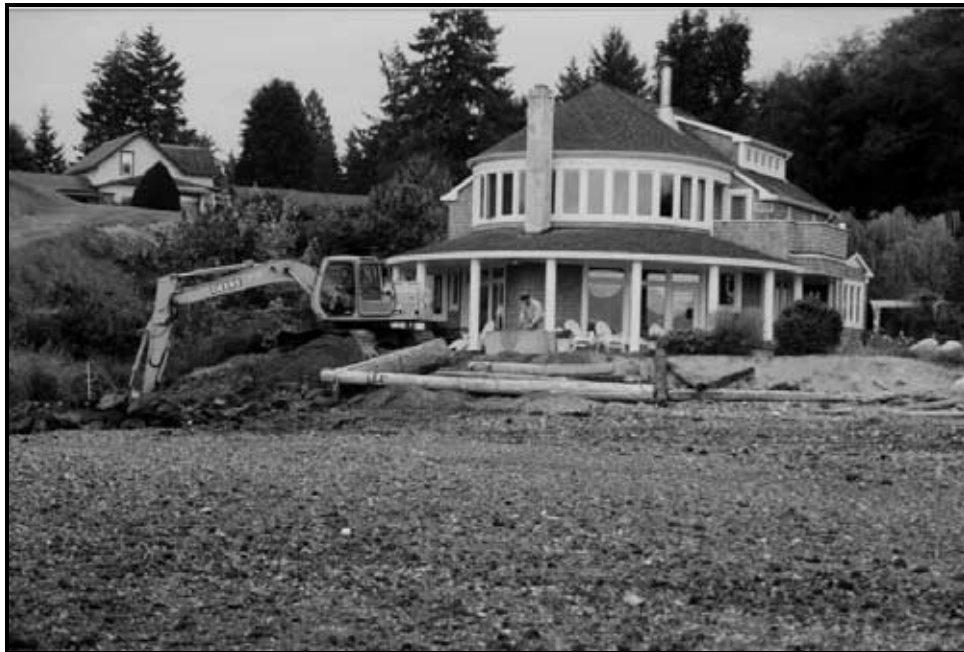
Figure 2. Construction. Note minimal setback and broad gravelly beach.
