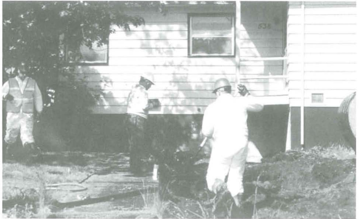
Remediation at the Everett Smelter site involves removing contaminated soil and sod from residential homes. Photograph taken by Dave South, Department of Ecology.
