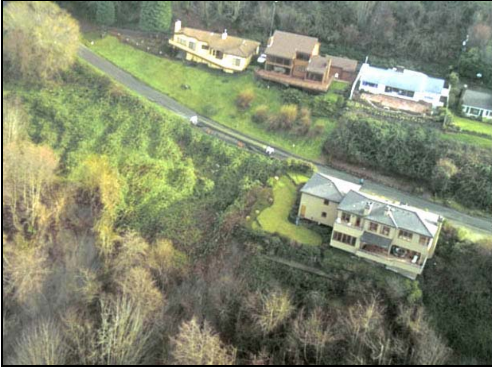
Figure 14. Landslide along Bonair Drive SW, above Alki Beach in West Seattle. Note scarp cutting downslope edge of road and through the lot in the foreground. [Photo: #4108_18, 1/2/1997]
