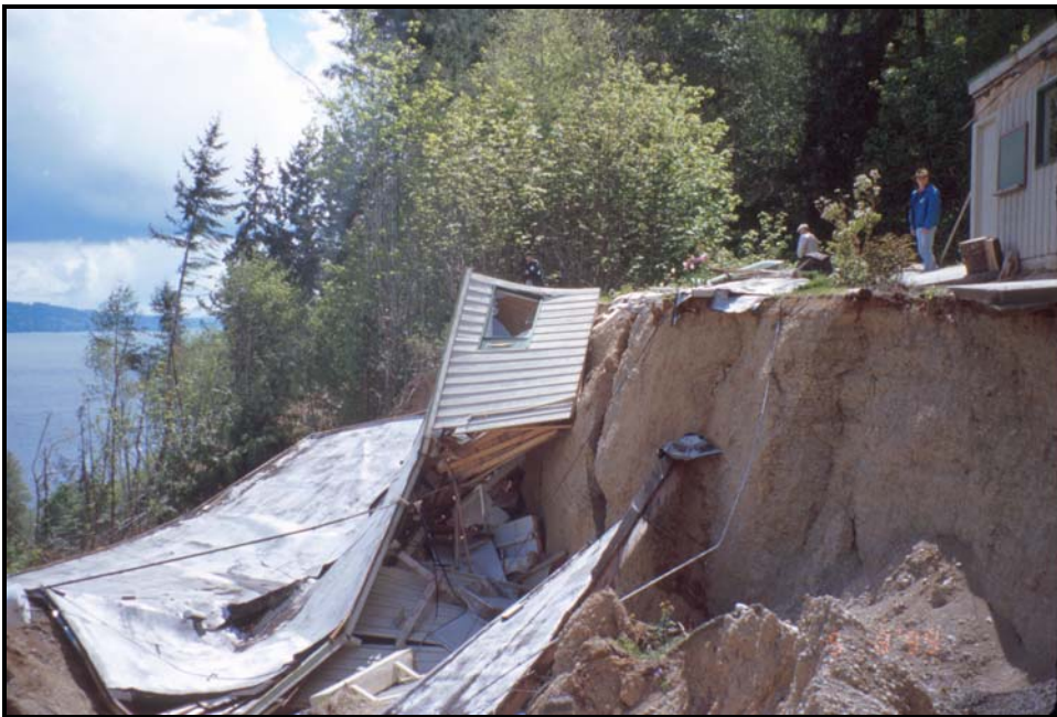
Figure 27. House destroyed at the headscarp of the Milepost 326 landslide. [Photo: 5/8/1999, #99-25-2]
