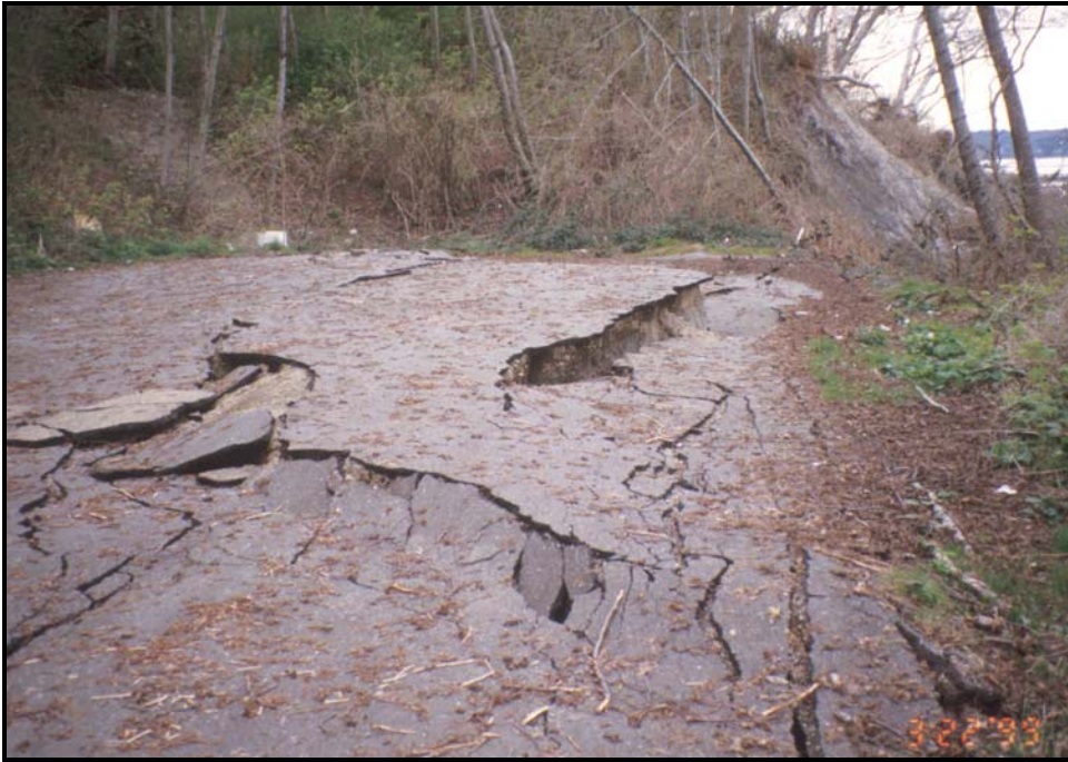
Figure 32. Disturbed asphalt at lower end of Killapie Beach Road. Shoreline is located to the right. [Photo: 3/22/1999, #99-11-25]
