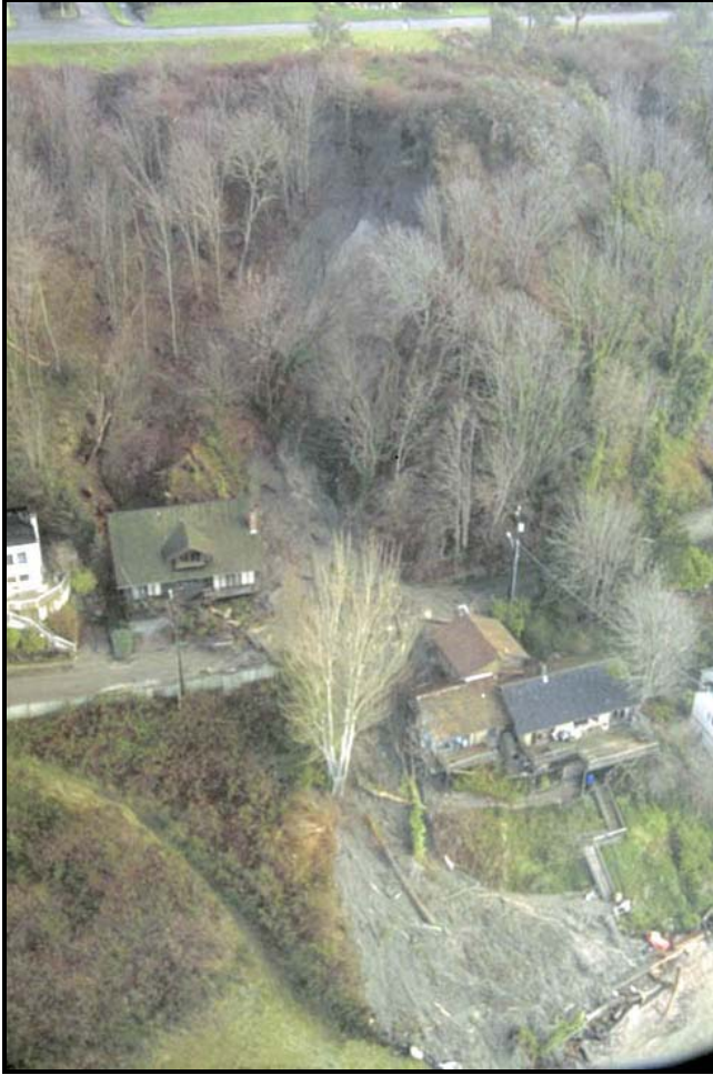
Figure 9. Debris flow downslope from a shallow landslide that occurred along Magnolia Bluff in Seattle during the 1996-97 Holiday Storm.
