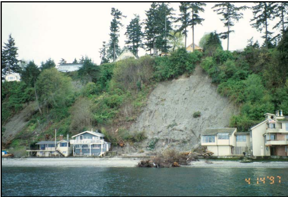
Figure 22. Site of destroyed Herron family home at Rolling Bay from the water. Vacant lot at left edge of photo is site of house destroyed by a landslide the previous winter. [Photo: 4/14/1997]
