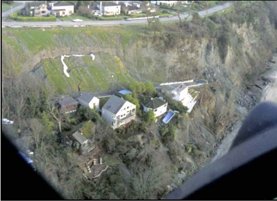
Figure 15. Aerial view of southeast end of Perkins Lane taken after the 96-97 Holiday Storm. Homes are located along a mid-slope bench. Note large failure in glacial till behind homes. [Photo: 1/2/1997, #4108_17]
