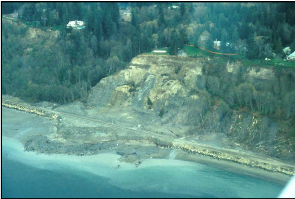
Figure 21. Woodway landslide from the air. Photo taken in late March, 1997. Prior relocation of the tracks waterward had left a broad trough at the base of the slope. The landslide filled this low trough, crossed the tracks, and formed a large point of land on the shoreline. [Photo: 3/30/1997, #97-22-17]
