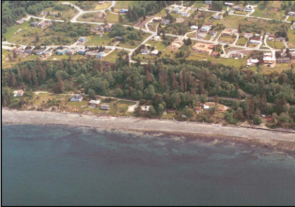
Figure 8. Aerial photograph of Ledgewood Beach landslide on Whidbey Island. Homes lower on slope are built on a deep-seated landslide, portions of which periodically reactivate resulting in damages to homes and roads. The toe of the landslide is located near sea level [Ecology, 5-5-199, ISL#0415]
