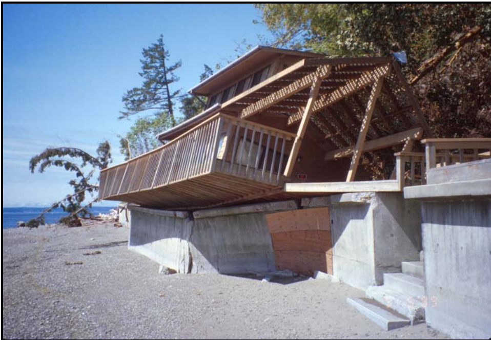
Figure 37. Beach cabin destroyed by landslide. Cabin was involved both in deeper movement of landslide and by debris avalanches from above. [ Photo: 5/5/1999, #99-24-1 ]
