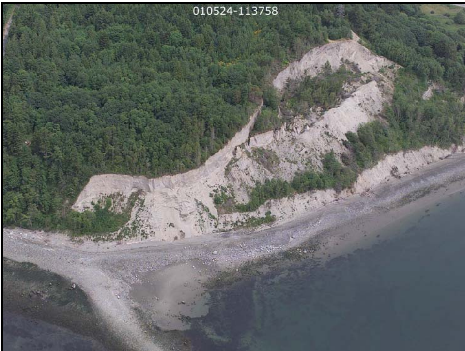
Figure 42. 2001 photograph of Point Roberts landslide. Area of 1999 failure can be seen on right half of image by comparing to 1994 photo (previous figure). [Ecology, 5/24/2001]
