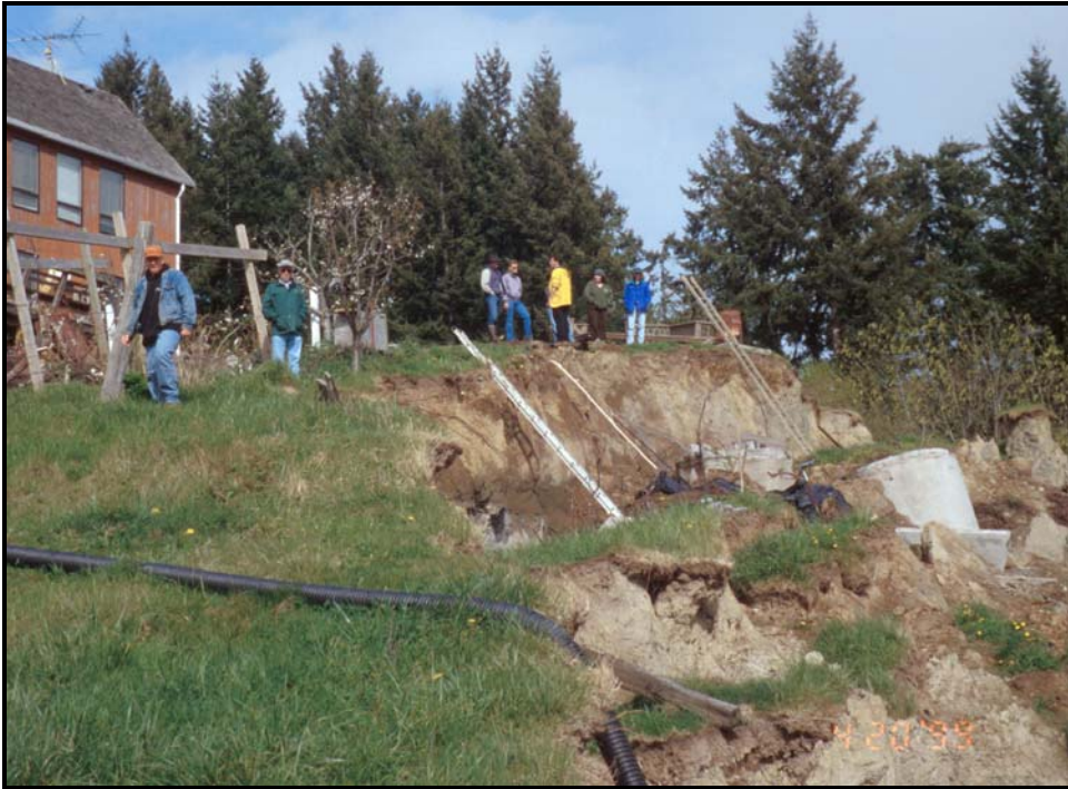
Figure 35. Headscarp of a large upper bluff slump overlooking Hood Canal, west of Termination Point. Original bluff edge was more than fifty feet farther to the right of the most recent scarp. Note septic tank and landscaping on the upper portion of the landslide mass. [Photo: 4-20-1999, #99-21-17]
