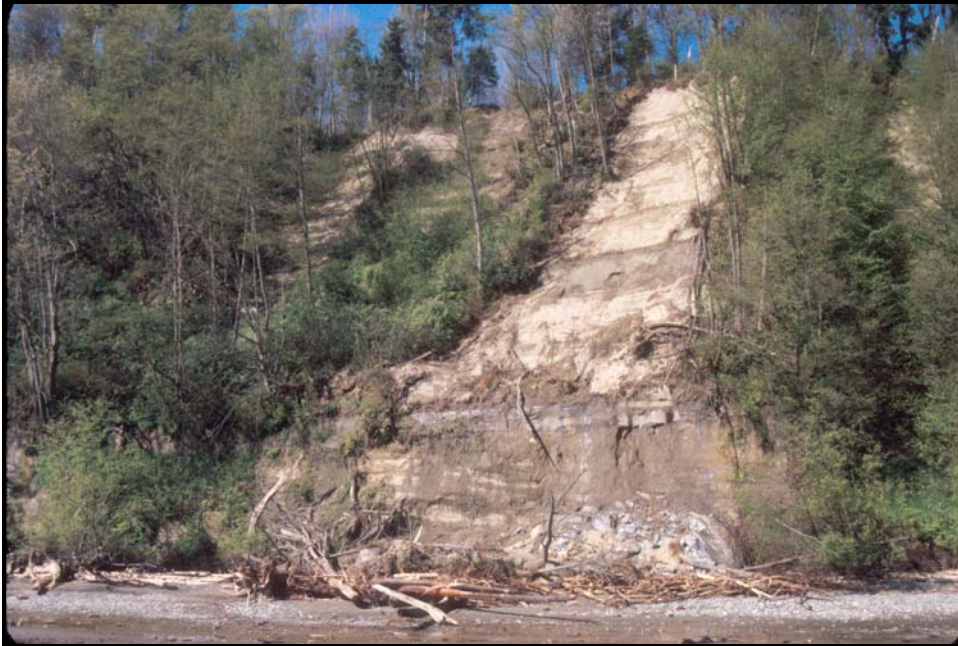
Figure 3. Shallow landslide exposing characteristic sequence of Puget Sound region geological units. The darker units in the lower part of the bluff consist of Lawton Clay and underlying Whidbey formation. Much of light-colored upper bluff consists of sandy advance outwash sediments (Esperance Sand). Vashon till caps the bluff. Note seepage along contact between outwash and Lawton Clay - this zone is likely where the landslide began. [Photo: Eglon area, Kitsap County, 1995, #95-17-7]
