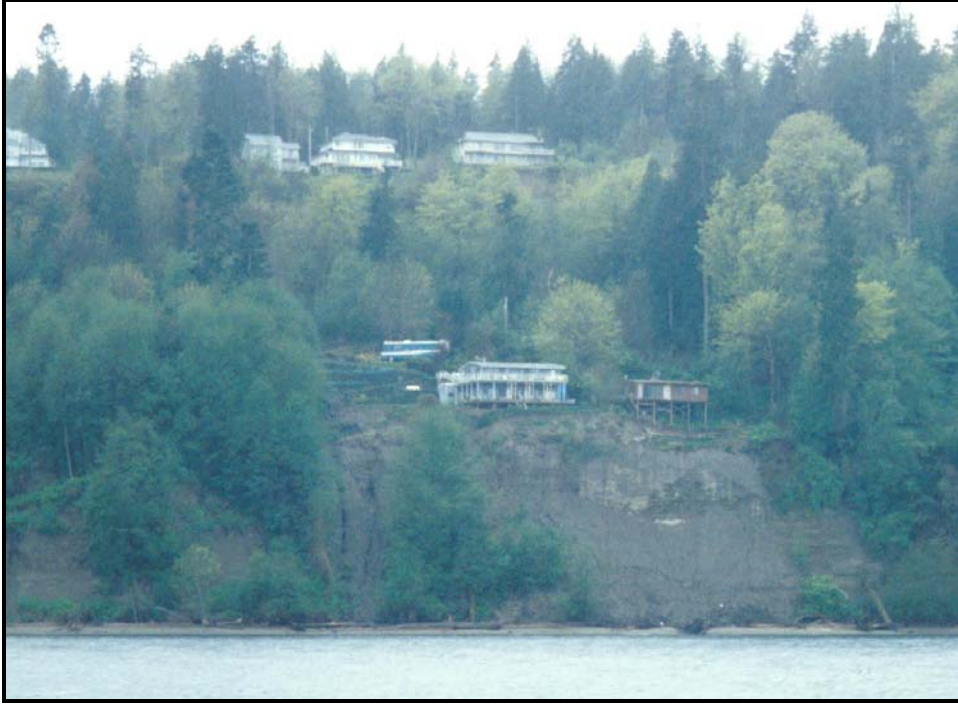
Figure 23. Mid-slope bench located along high bluffs north of Kingston and Apple Cove Point. Home in foreground was impacted by 1996-97 landslides. [Photo: 4/14/1997, 97-30-18]
