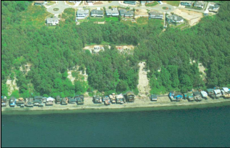
Figure 43. The Salmon Beach community in Tacoma is built on piles at the base of a steep, unstable bluff. A large landslide developed on the slope above this community following the February, 2001, Nisqually Earthquake - see Appendix. [ Ecology , 5/16/1992, PIE#0116]
