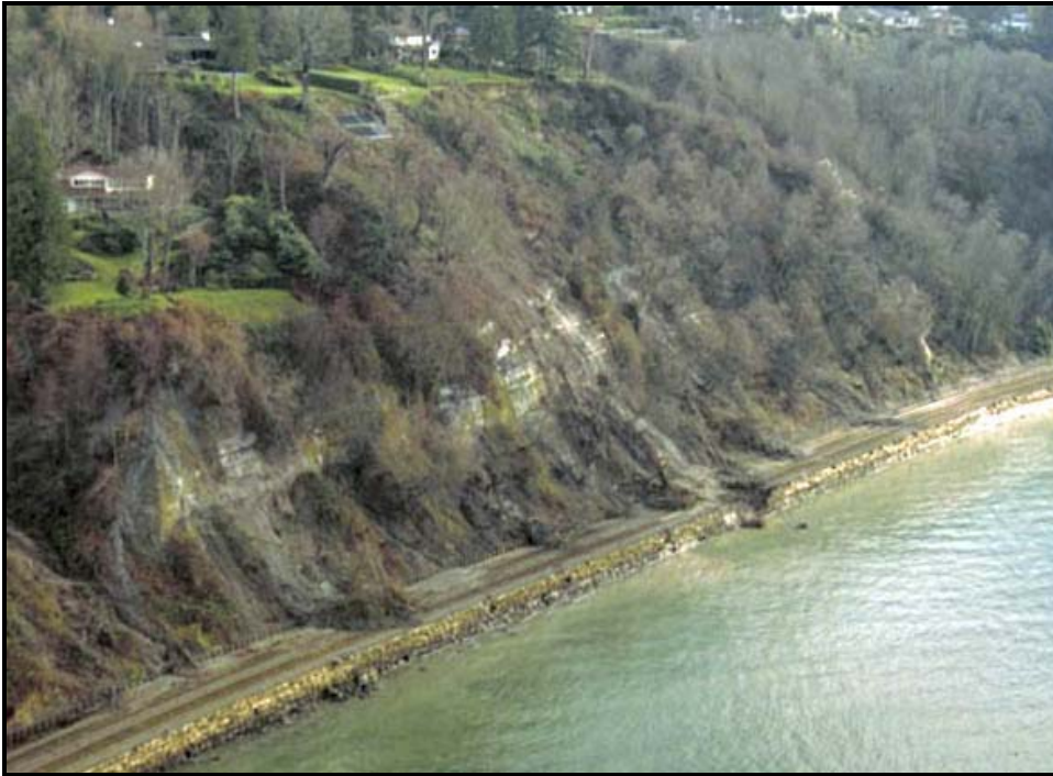
Figure 19. Aerial view of landslides over railroad tracks north of Seattle. [Photo: 1/2/1997, #4108_19]
