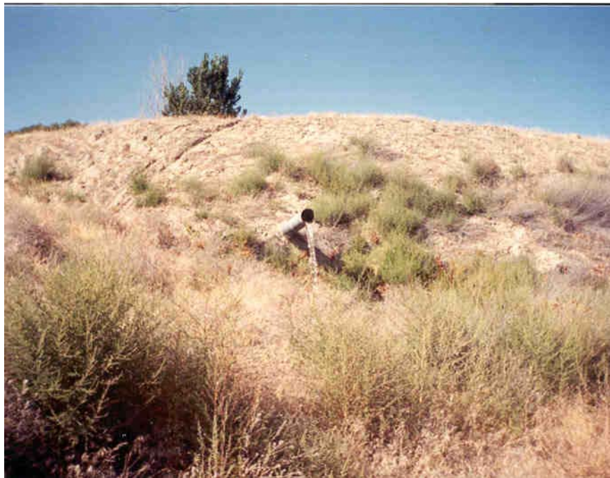
Photo 11: Irrigation water is being drained out of the Ringold formation to prevent slope failure. Location is near photo 10.
