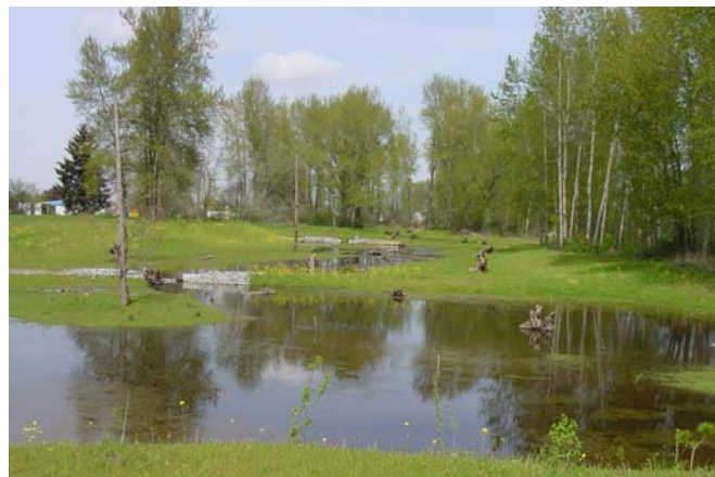
The Lake Tapps Parkway Mitigation Site after construction in April 2001.
