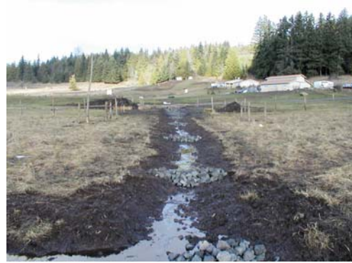
Drainage Ditch - before
