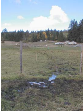
Drainage Ditch – after
