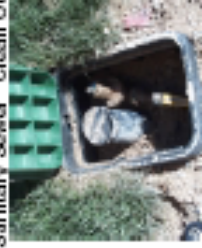
Sanitary Sewer "Clean Out"
