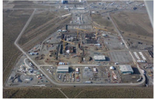
Hanford's Tank Waste Treatment Plant under construction
