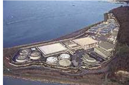
Wastewater Treatment Plant
