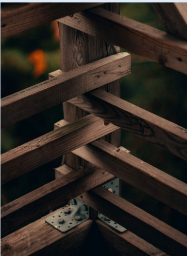
Figure 3: Treated wood may be reused in normal treated wood applications, such as fences.
