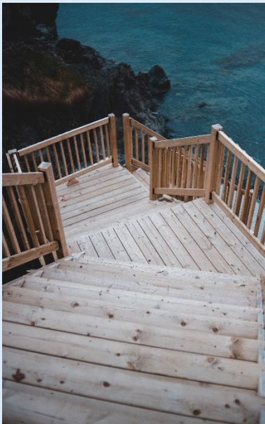
Figure 8: Treated wood is often used outdoors.
