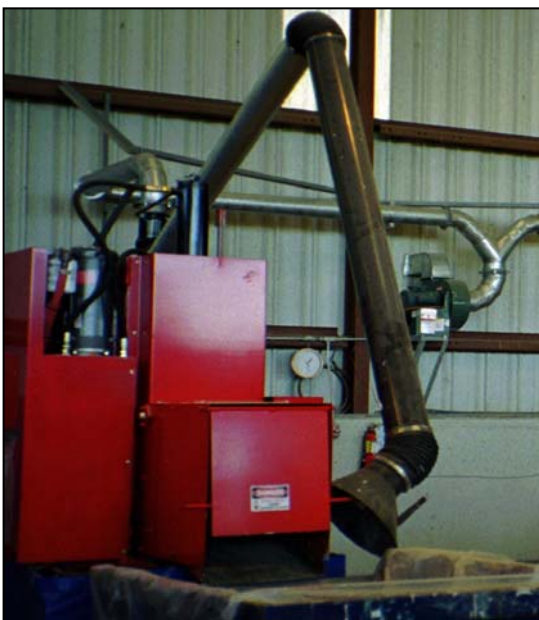
HHW Spot Ventilation at Cowlitz County
