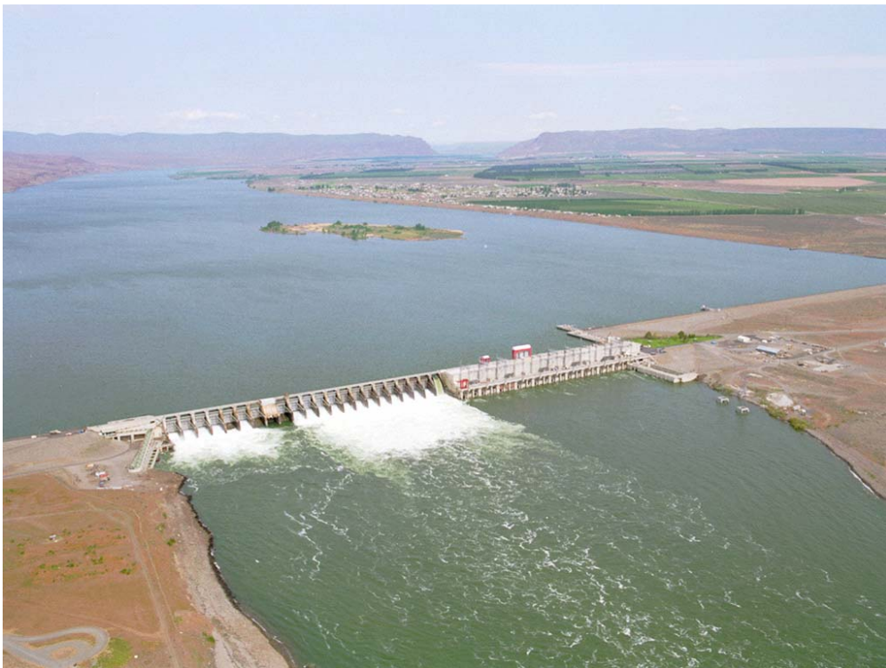
Figure E-7. Priest Rapids Dam
