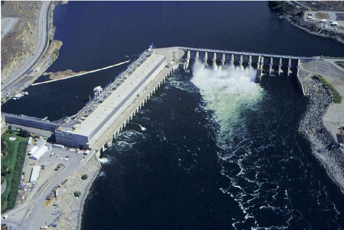
Figure E-4. Rocky Reach Dam
