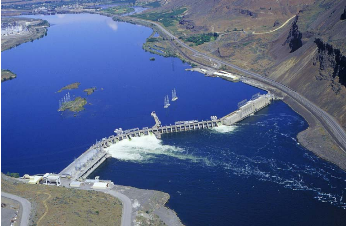
Figure E-5. Rock Island Dam
