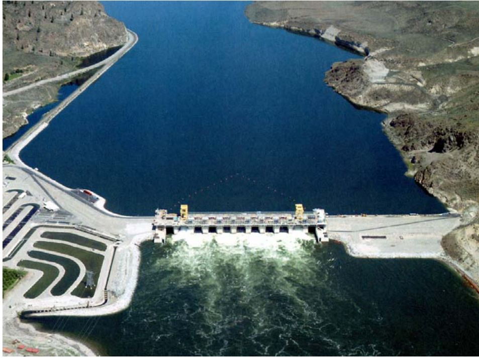
Figure E-3. Wells Dam
