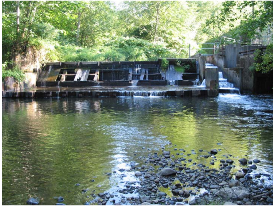
Figure 5. Issaquah Salmon Hatchery water-supply intake dam and fish ladder on Issaquah Creek near Wildwood Apartments.
