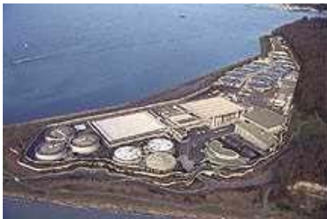
Wastewater Treatment Plant
