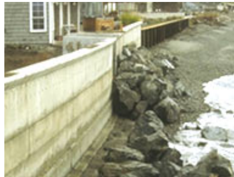
Bulkheads increase wave action and scouring of the beach
