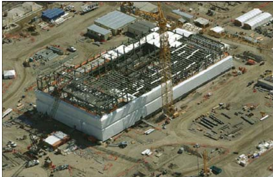
Hanford's Tank Waste Treatment Plant under construction
