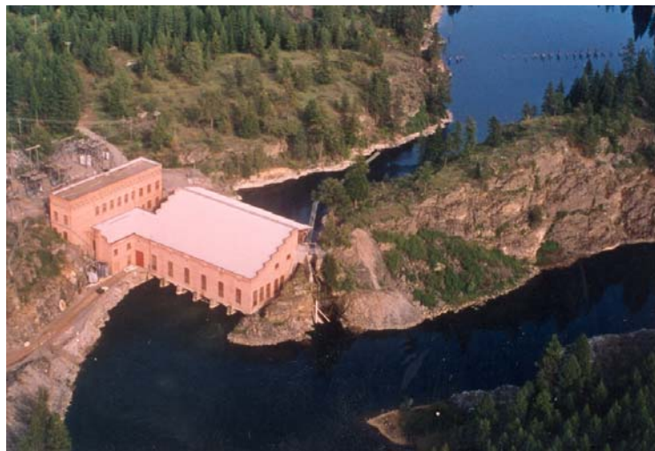
Middle Channel with Powerhouse
