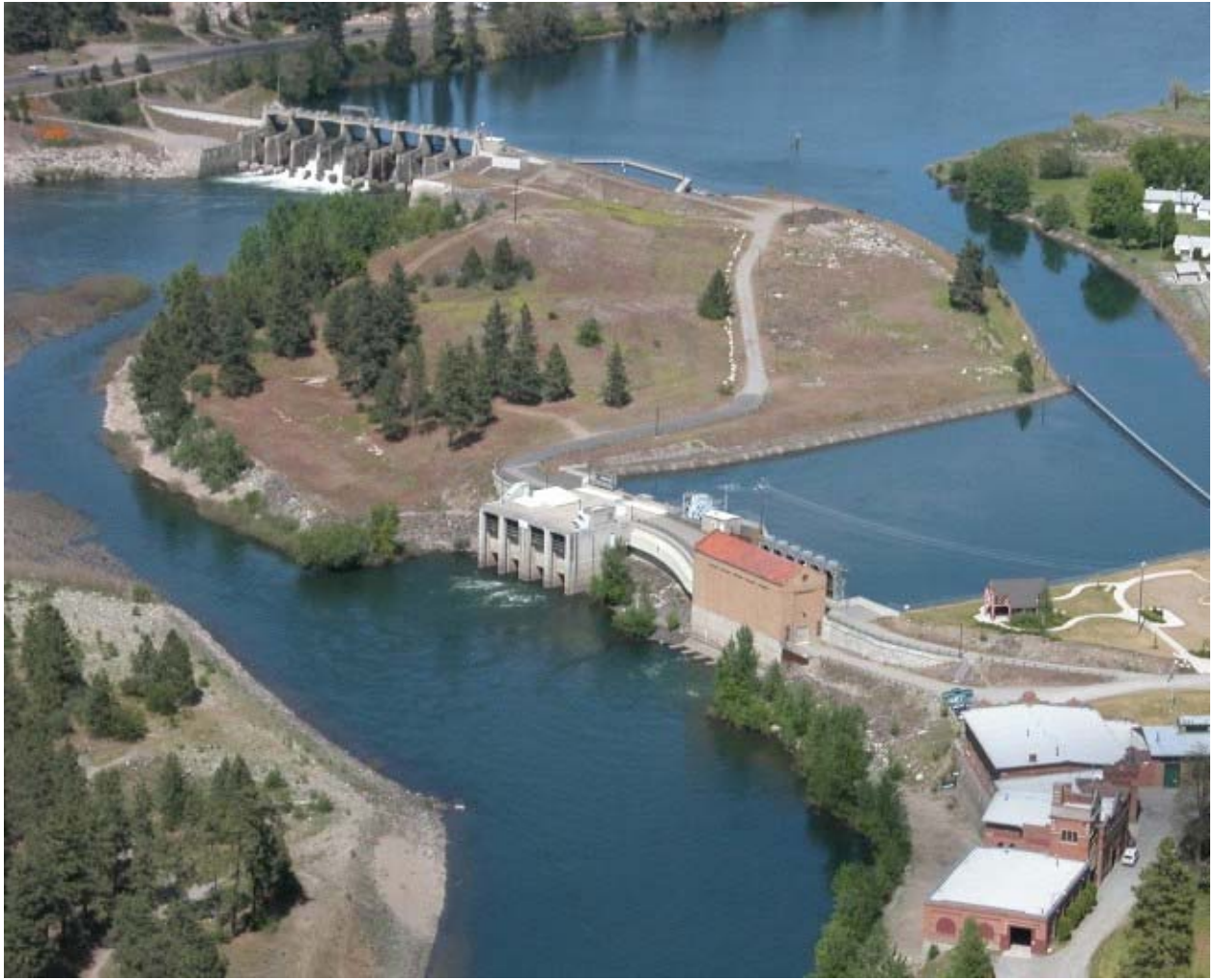
Figure 3. Upriver Dam (Photograph Courtesy of City of Spokane)
