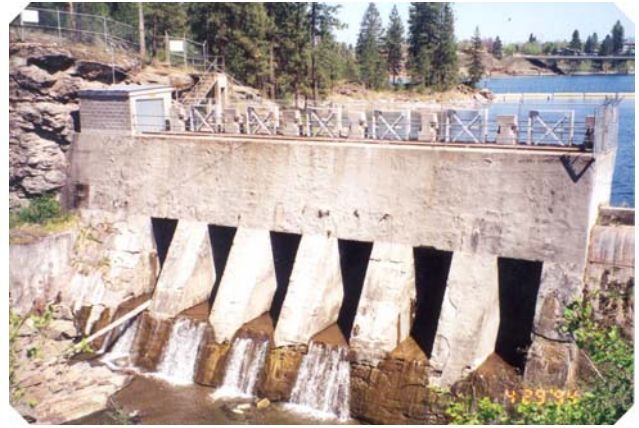
South Channel without Spill
