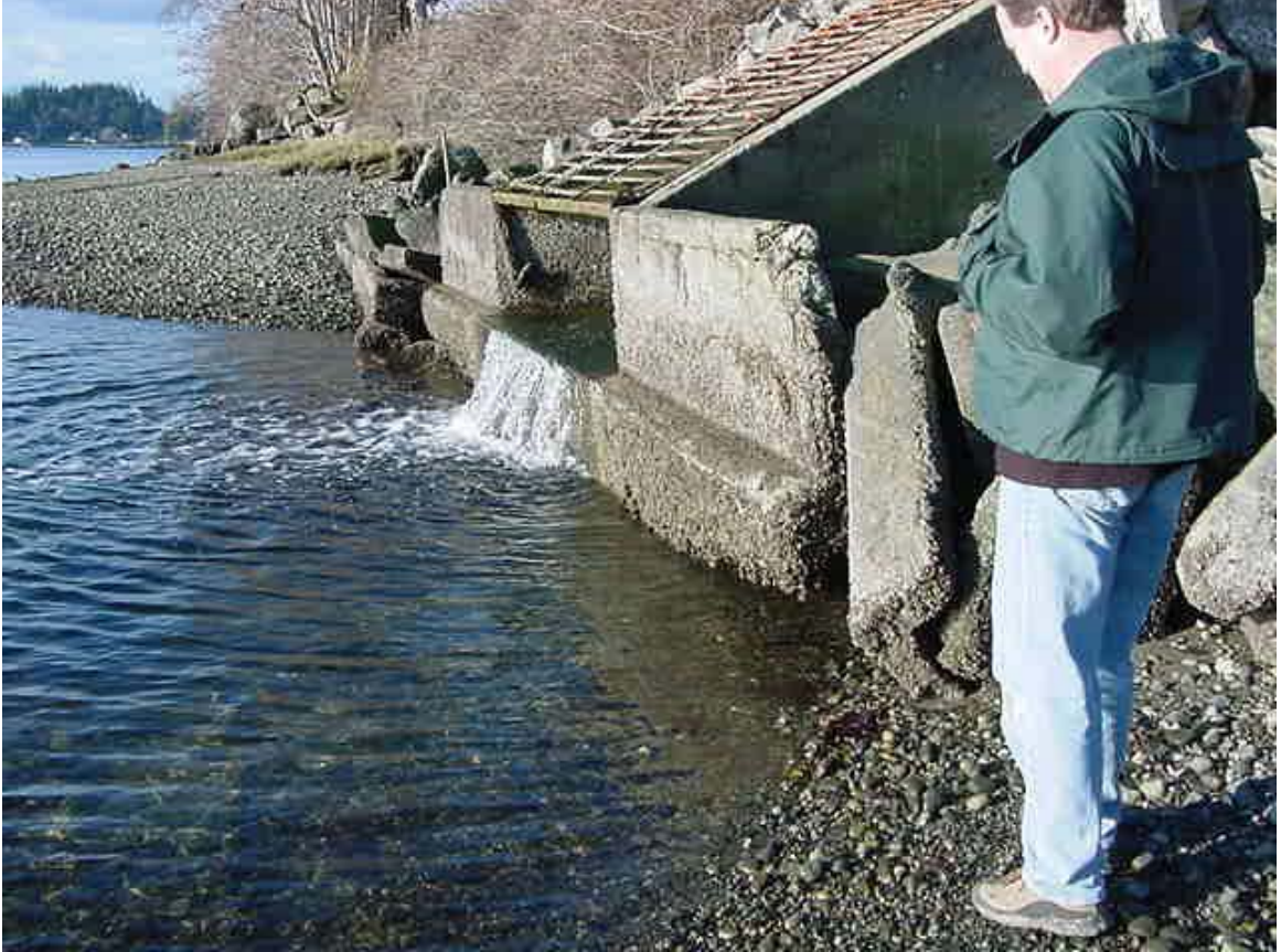
Photo 7. Storm water outfall discharging from East Bremerton into the Port Washington Narrows (Project ENVVEST File Photo).
