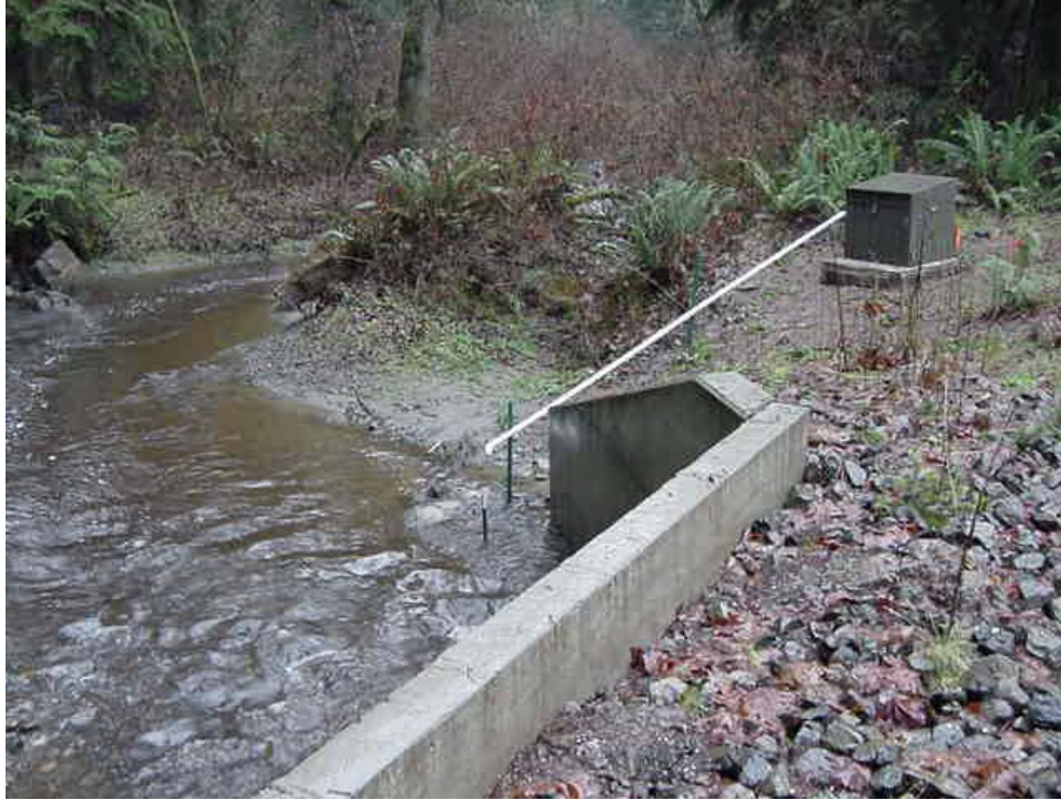
Figure 4-2. Barker Creek Water Quality Sample Station, Showing Automated Sampling System Enclosure and Sample Pipe
