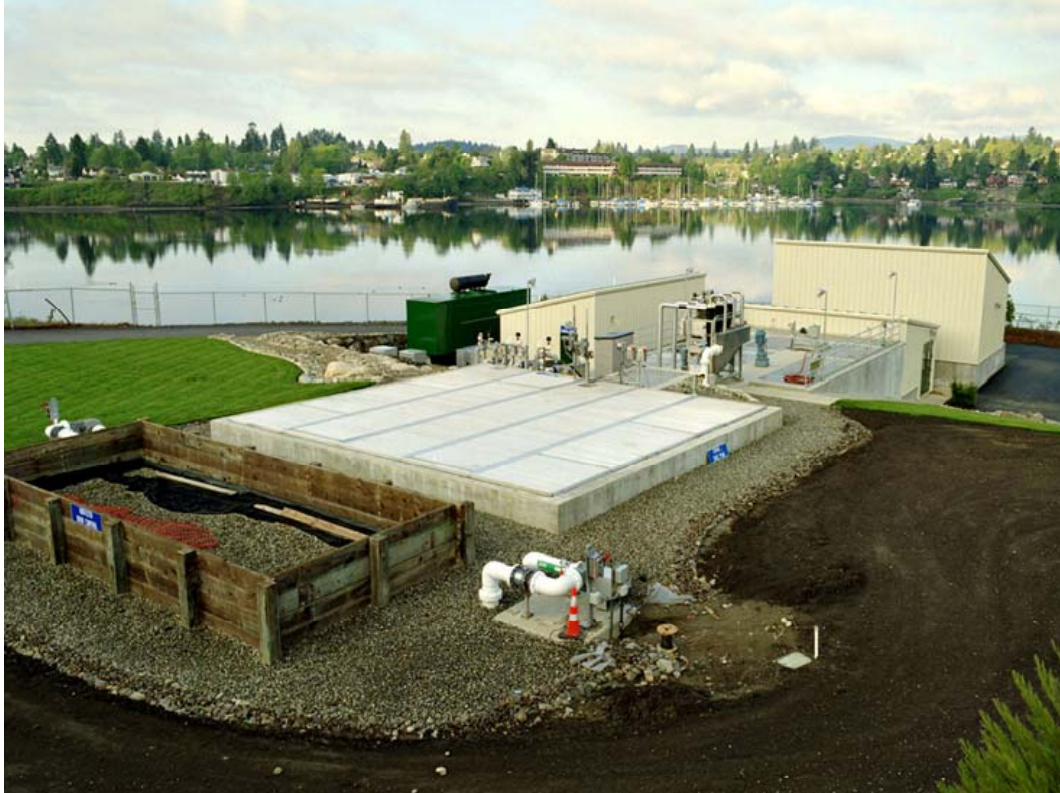
Photo 9. The Eastside Treatment Facility on the Port Washington Narrows in Manette. The facility was built by the City of Bremerton to control storm water runoff from East Bremerton. Completed in December 2001, the facility can efficiently treat 14 - 20 MGD, clarifying wastewater to meet the water quality standards and disinfecting the treated water with ultraviolet light. (Photo by City of Bremerton)
