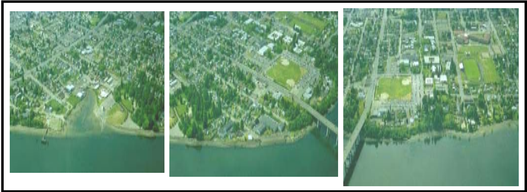
Figure 4 Aerial Photographs of Dyes Inlet West Shoreline going south to north (upper left to Lower right).
