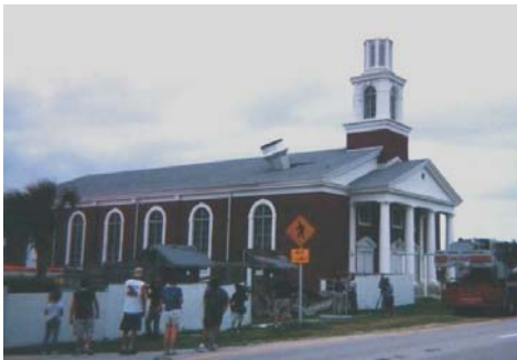
This steeple was knocked upside-down by a hurricane.
