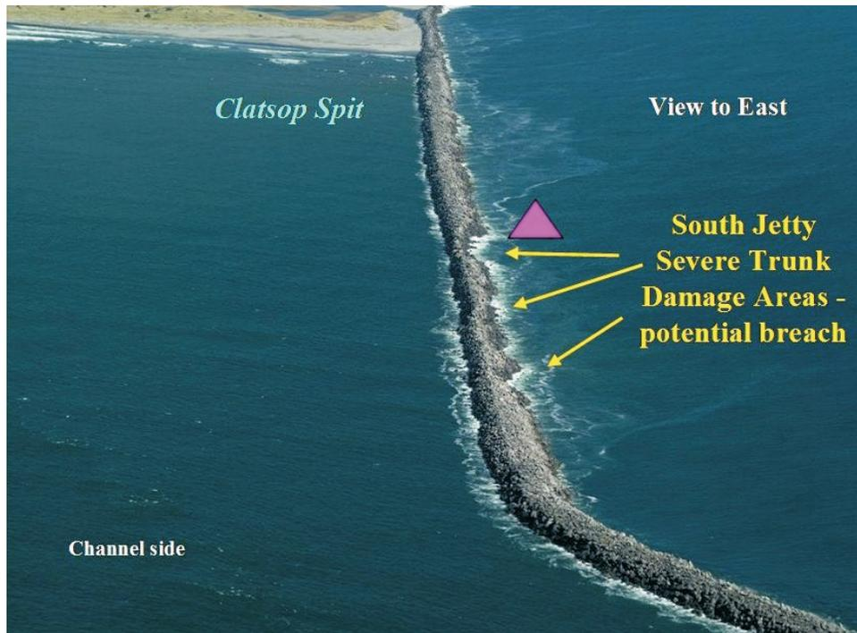
Fig. 45. Photograph of jetty section east of the “knuckle” taken September 11, 2002 (courtesy of Hans R. Moritz).
