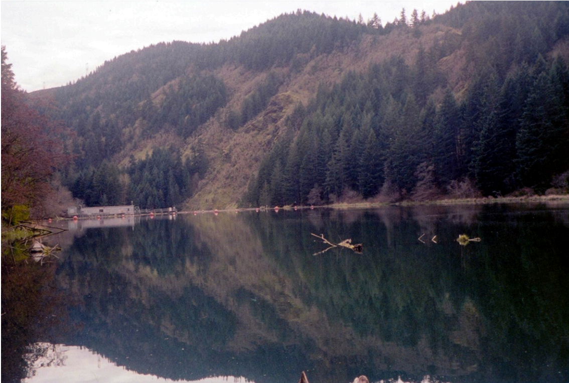
Figure 4.10-1. Looking south toward dam (about 200 feet north of dam) part 1 of 3 photo panorama
