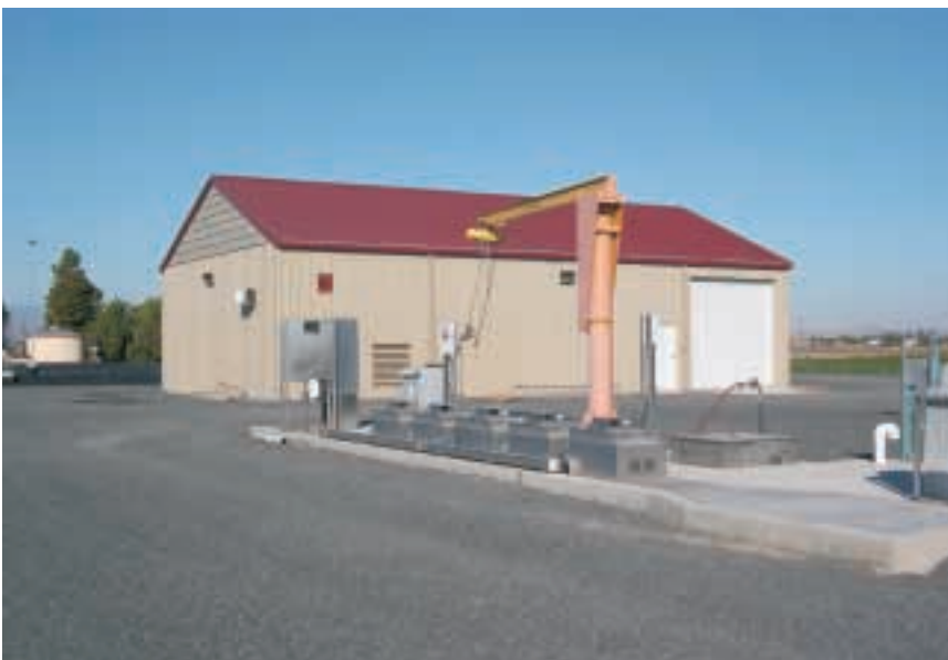
Advanced treatment and control building. UV channel in foreground. Ecology photo
