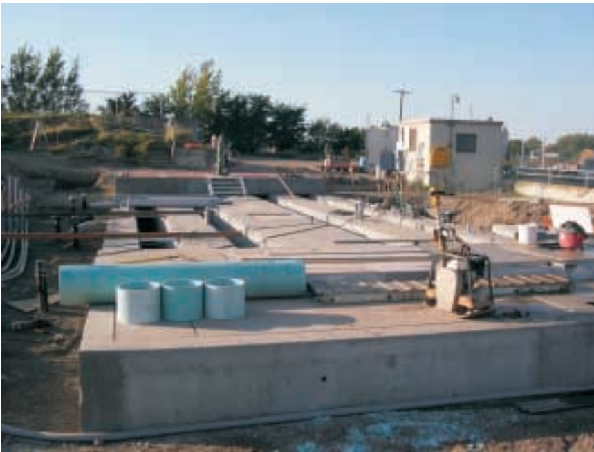
Construction of the UV channel at Walla Walla. Ecology photo
