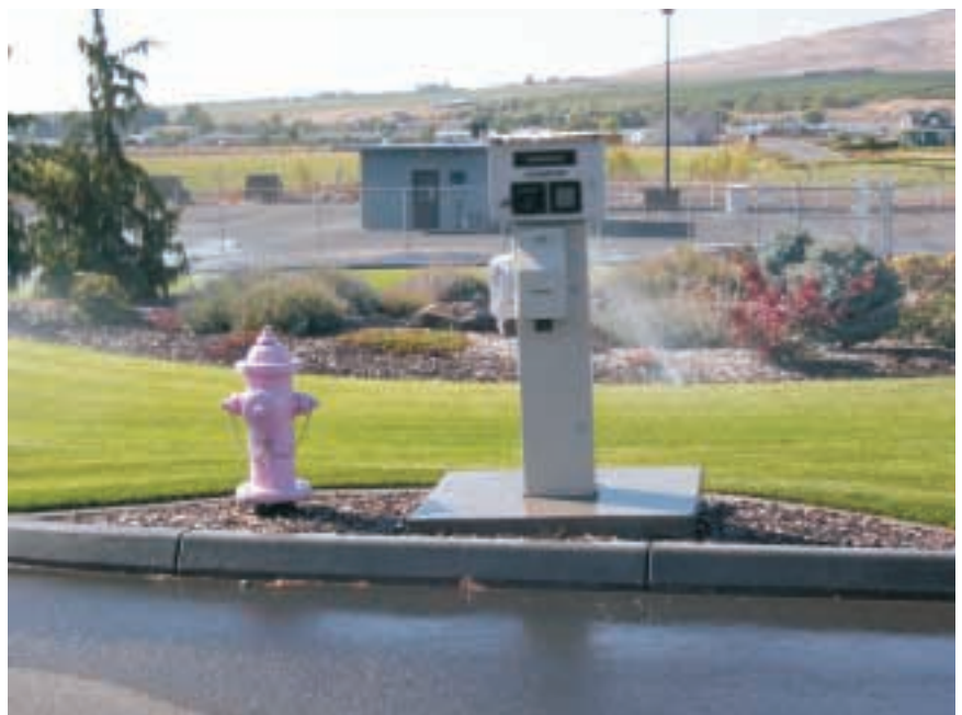
Reclaimed water hydrant and water meter. Ecology photo
