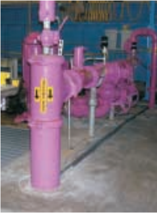
Purple pipes at Medical Lake treatment facility pump the Class A water to Medical Lake and Deep Creek. Ecology photo
