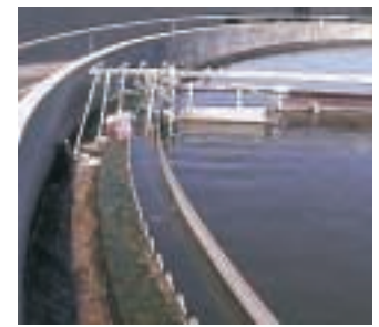
The clarifier removes solids following secondary treatment. Ecology photo
