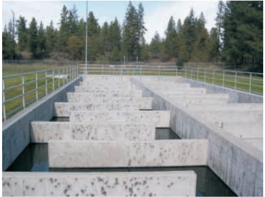
Chlorine disinfection units at Cheney facility. Ecology photo
