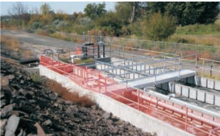
Re-aeration of water for discharge to Garrison Creek. Ecology photo
