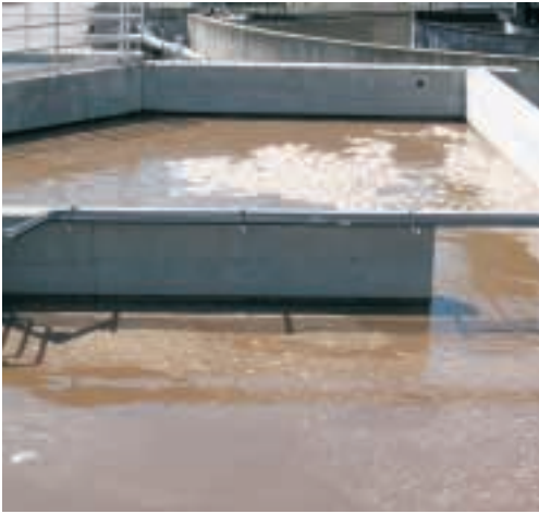
Wastewater secondary treatment at the Snoqualmie oxidation ditch. Ecology photo
