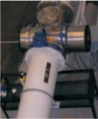
College Place's medium pressure ultraviolet disinfection unit. Ecology photo
