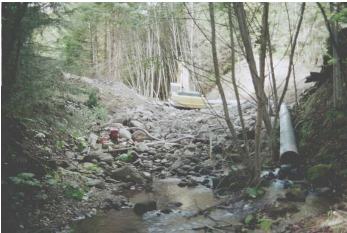
Figure 3: Culvert Removal from Slide Creek, Greenwater River
